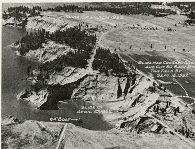
Figure 2.21. Reed Terrace area, Lake Roosevelt, Washington, August 1, 1952, after landslide of April 10, 1952 (2.79, 2.182).
