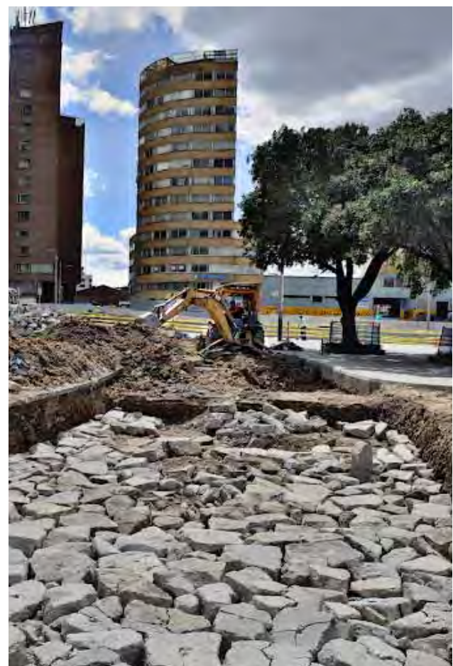
Bogota, Colombia. Excavation for improving public roads. © Victor Alfonso González
