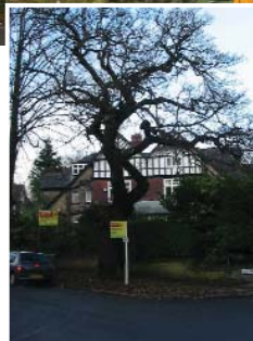
Eltonhurst and Oakfield on North side of St. Mary's Road are a striking pair of semi-detached houses designed in 1885
