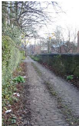
Stone setts and wall (right) between Chapel Road and Back Shelbroke avenue are important historical and visual features.
