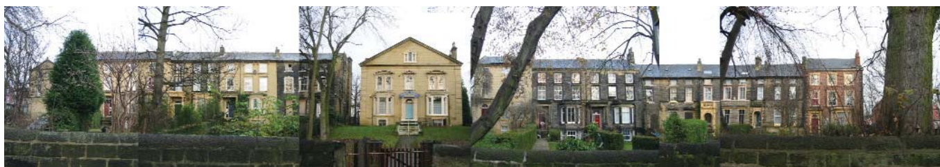
Newton Grove frontage to Harehills Avenue
