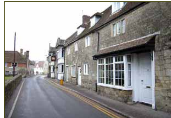
Figure 17 Attractive group of mainly seventeenth century cottages, Church Street (fronting the church and churchyard)
