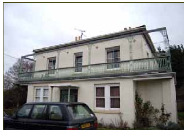
Figure 19 Balcony and veranda to Bridge House
