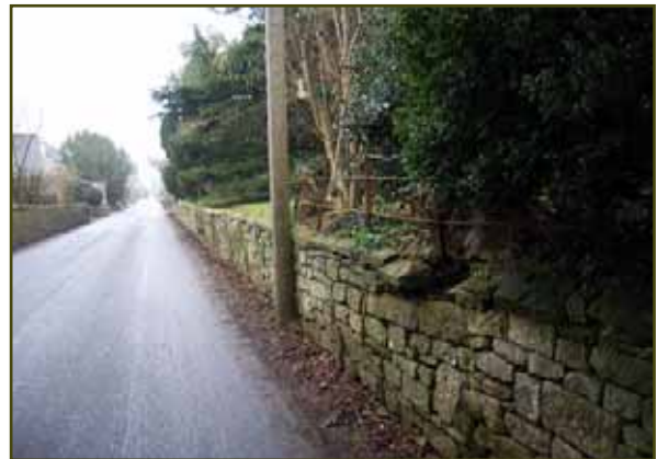
Figure 1 'Dry stone' boundary walls to Hindon Lane
