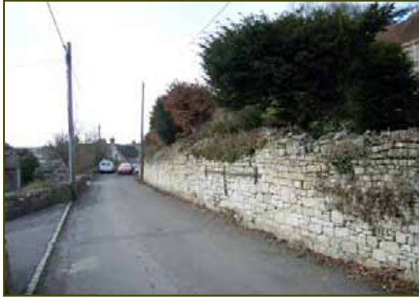
Figure 9 Boundary wall to The Grange, Vicarage Road
