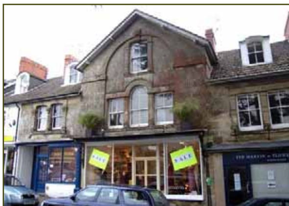
Figure 25 Well detailed groups of purpose built shops and flats above, The Square
