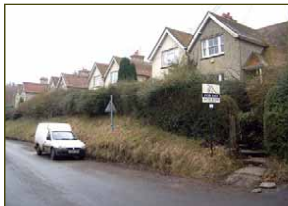
Figure 26 Estate type cottages in pairs form important part of the entrance to the conservation area (Hindon Lane)
