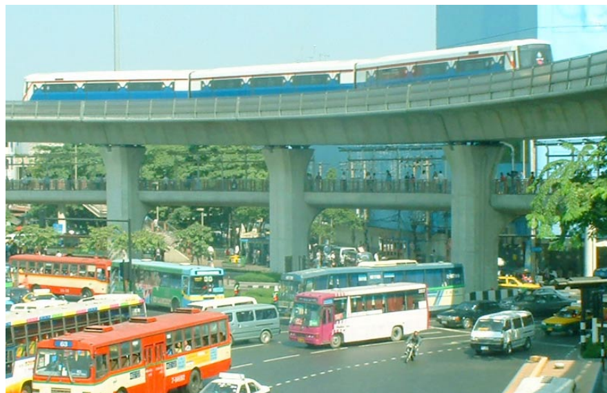
Fig. 21 ▼ Victory Monument, Bangkok. BTS trains run on dual tracks, carried on a 9 metre wide viaduct, supported on single box viaduct girders, each 12 metres above the road level.
