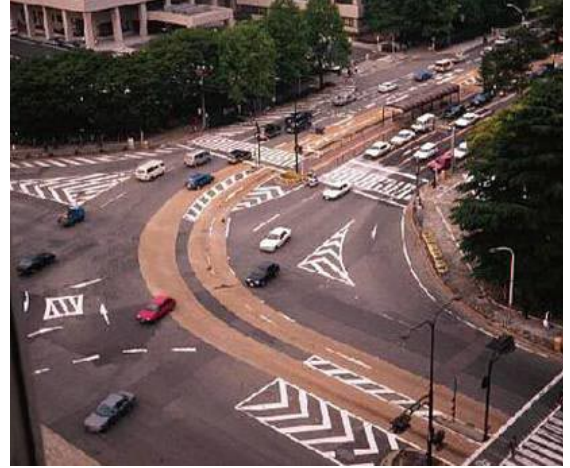
Fig. 9 ▲ Nagoya, Japan, marks the bus lanes with a coloured road surface. Courtesy of John Cracknell, TTC, and the US Transportation Research Board.
