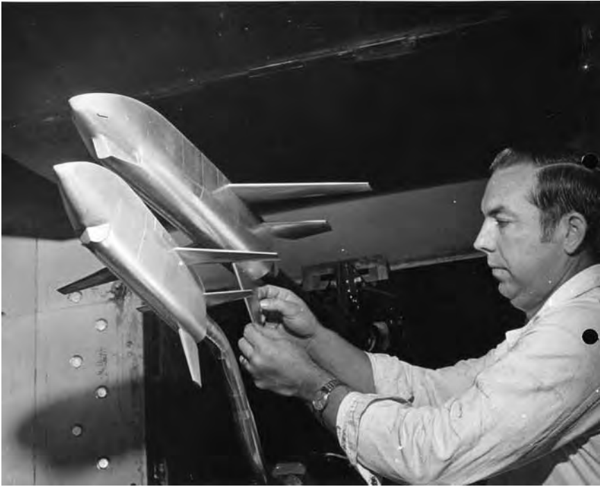
When the concept of a space shuttle emerged in the latter 1960s, NASA envisioned it as a two-stage, fully reusable vehicle with both parts landing on a runway. This wind tunnel model represented the "DC-3" concept developed by Max Faget at the Manned Spacecraft Center (renamed the Johnson Space Center in 1973). NASA.
