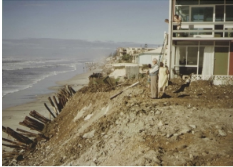
Figure 4.4: Severe beach erosion at Palm Beach during 1967 (EPA photograph).
