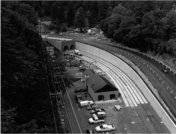
Westside MAX tunnel east portals, 1997
