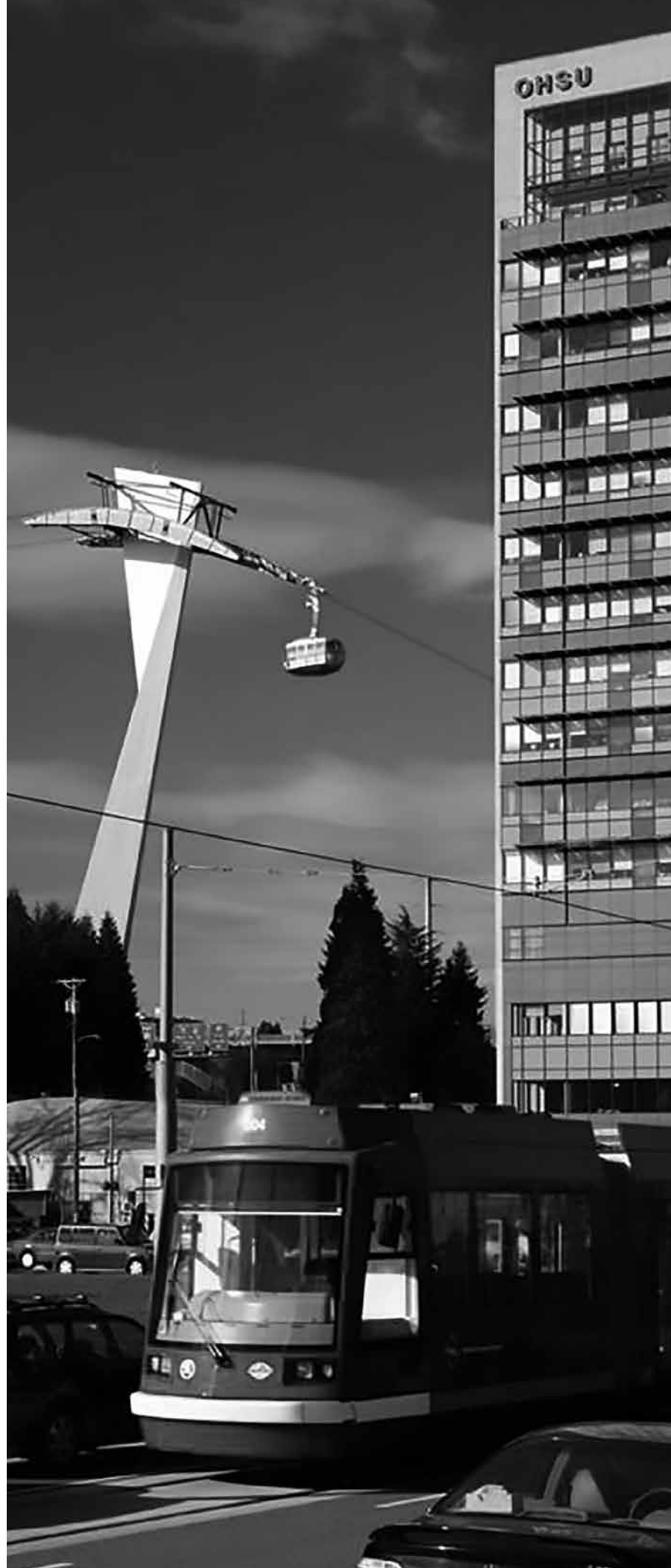
Portland Aerial Tram at Oregon Health and Science University building in South Waterfront, 2007
