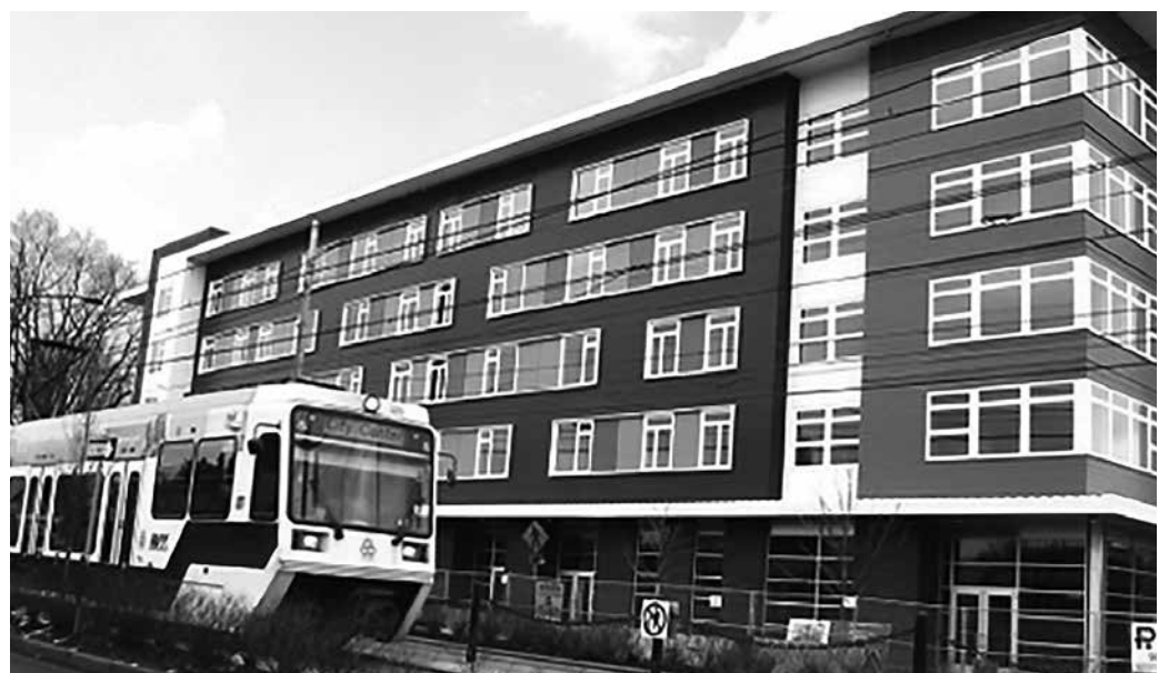
Patton Park Apartments on Interstate Avenue, a TriMet collaboration with REACH Community Development, 2009
