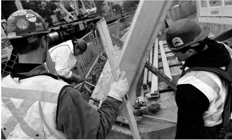
Construction workers on MAX Green Line, 2009
