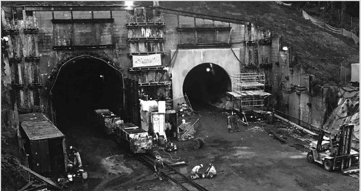
Westside MAX tunnel east portals, 1995
