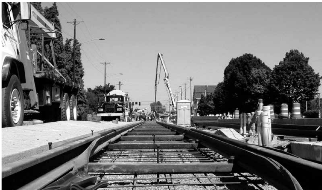
Laying tracks on North Interstate Avenue, 2002
