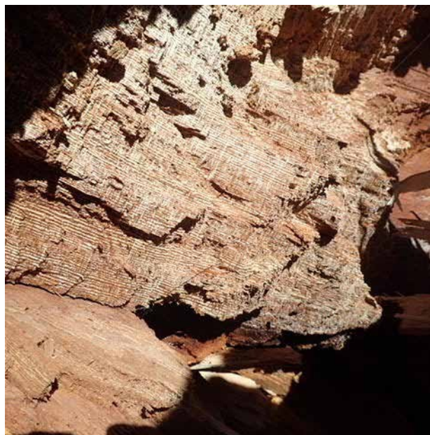
Photo 4. The decayed wood of Fig has distinctive brown stripes.
