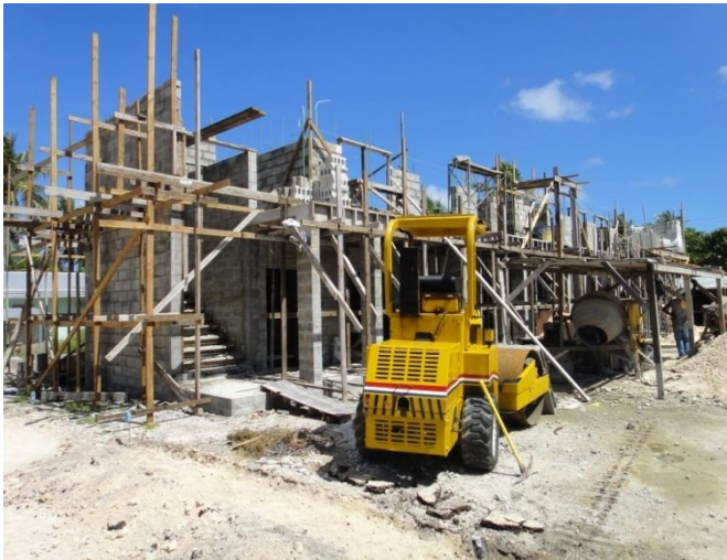
Ongoing construction at Rairok Elementary School
