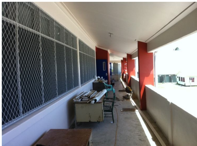
Ebeye Elementary School Maintenance Project
