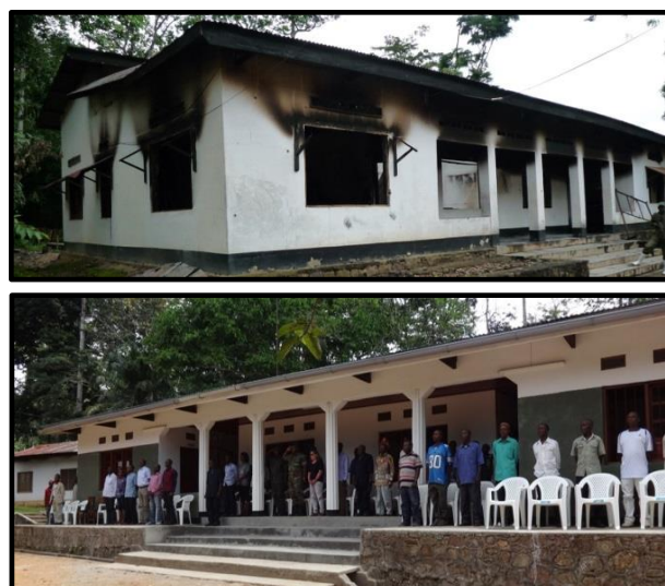
Figure 15. ICCN office building in Okapi Wildlife Reserve headquarters, burnt-out following rebel attack in June 2012 (top) and rebuilt in March 2014 (bottom). © OCP 2015
