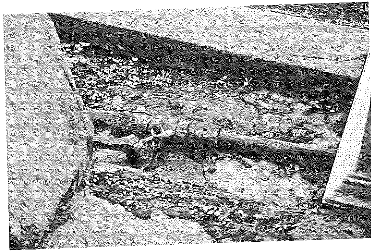
Figure 11.6. Bronze stopcock on a lead pipe supplying an ornamental fountain in the peristyle of the House of the Vettii, Pompeii. (Photograph by: A. I. Wilson.)
