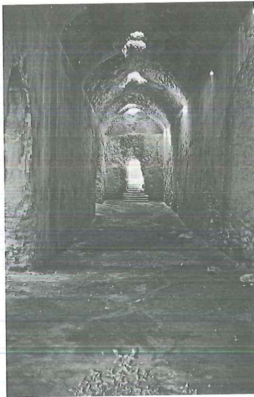
Figure 11.7. One of seven parallel vaulted chambers in the large reservoir cisterns at Oudhna (ancient Uthina) in Tunisia. (Photograph by A. I. Wilson.)
