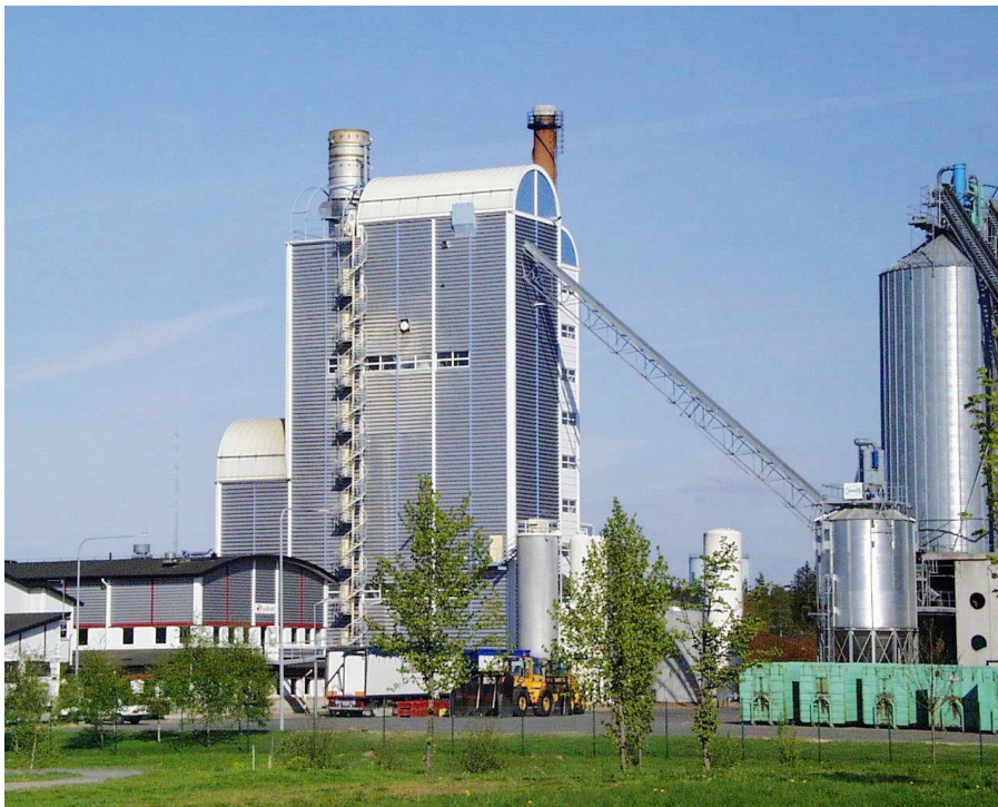
Värnamo (Sweden), a plant for biofuel-fired combined heat and power generation based on pressurized gasification
