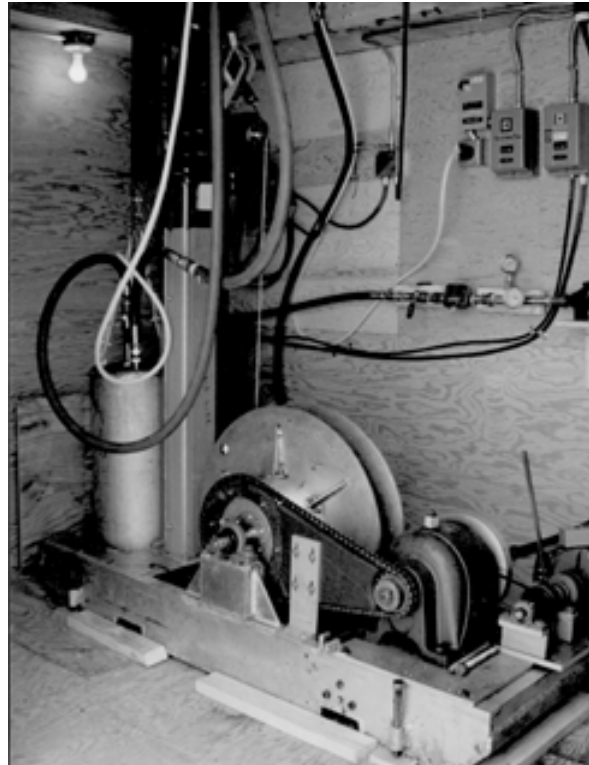
Figure 11. Hot-water drill used to drill second access hole to the SPWW.
