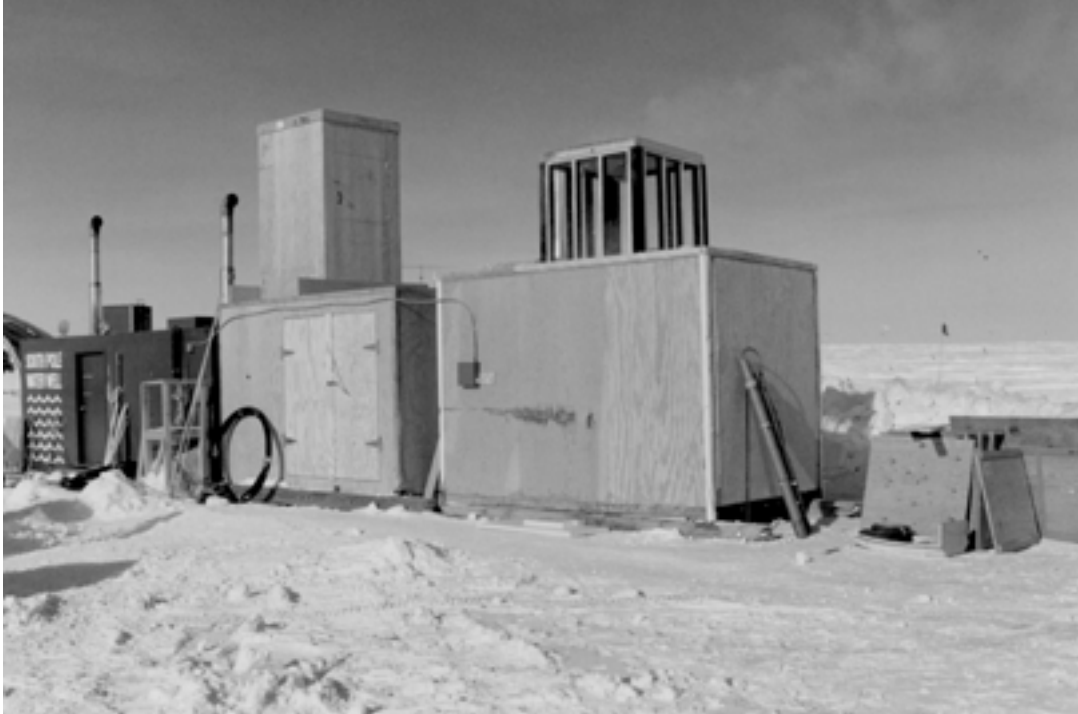
Figure 10. Work space at the SPWW, consisting of a winch room directly over the access hole and an adjoining laboratory.
