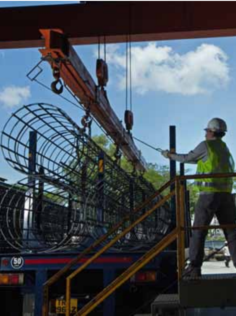
Safe loading at NatSteel, Singapore.
