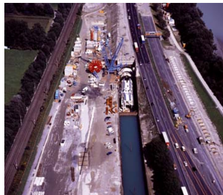
Construction works on Unterinntal Route
