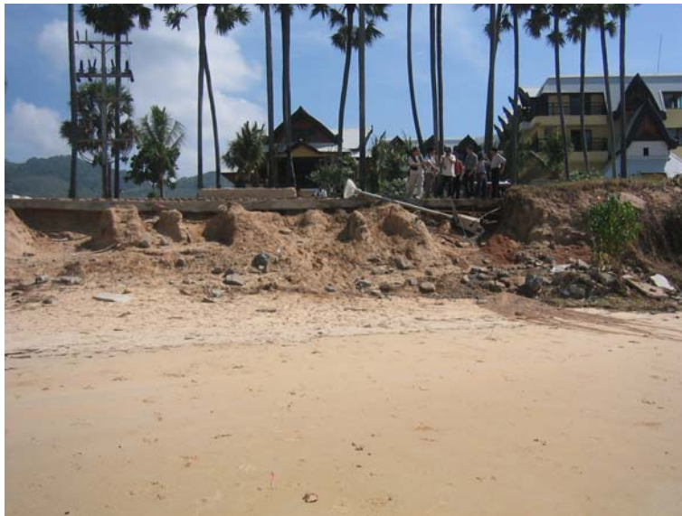
Photo 4.12 Karon Beach. The high road reduced the tsunami by acting as seawall
