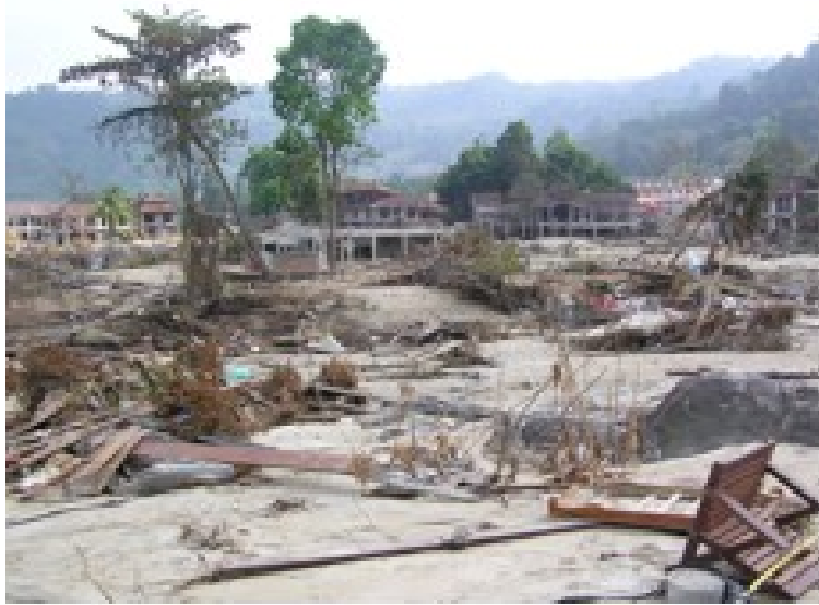
Photo 4.8 Heavily damaged hotels in Khao Lak
