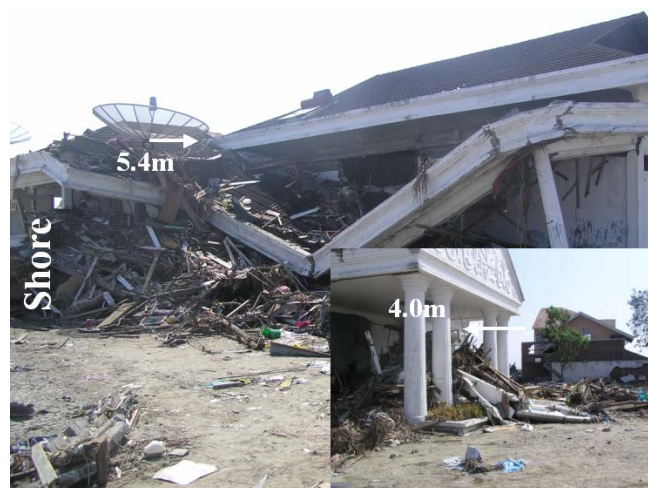
Photo 2.5 Partially damaged family house about 1.3 km inland in Banda Aceh. Left side is shore and right side inland. Numerals indicate inundation depths.
