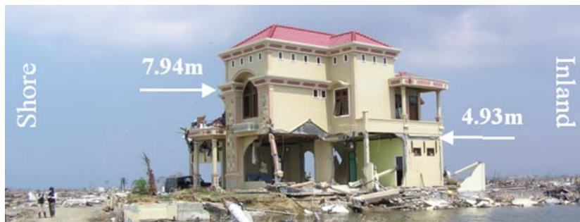
Photo 2.4 Partially damaged family house located about 0.9 km inland in Banda Aceh. Left side is shore and right side inland. Numerals indicate inundation depths.
