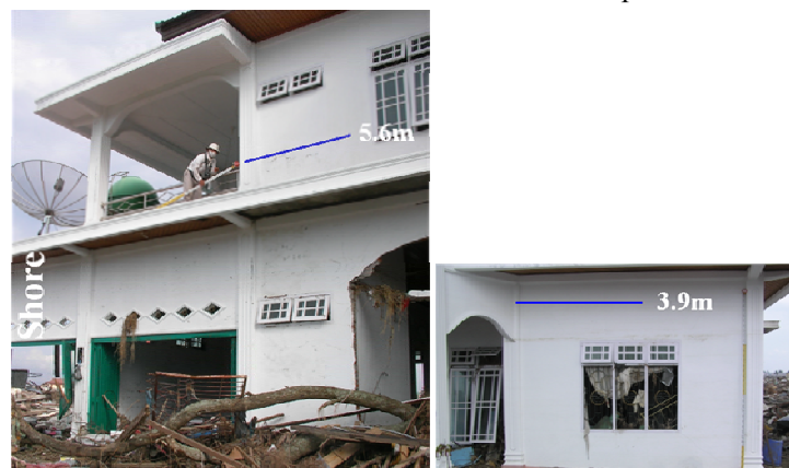
Photo 2.6 Partially damaged family house about 2.3 km inland in Banda Aceh. Left side is shore and right side inland. Numerals indicate inundation depths.
