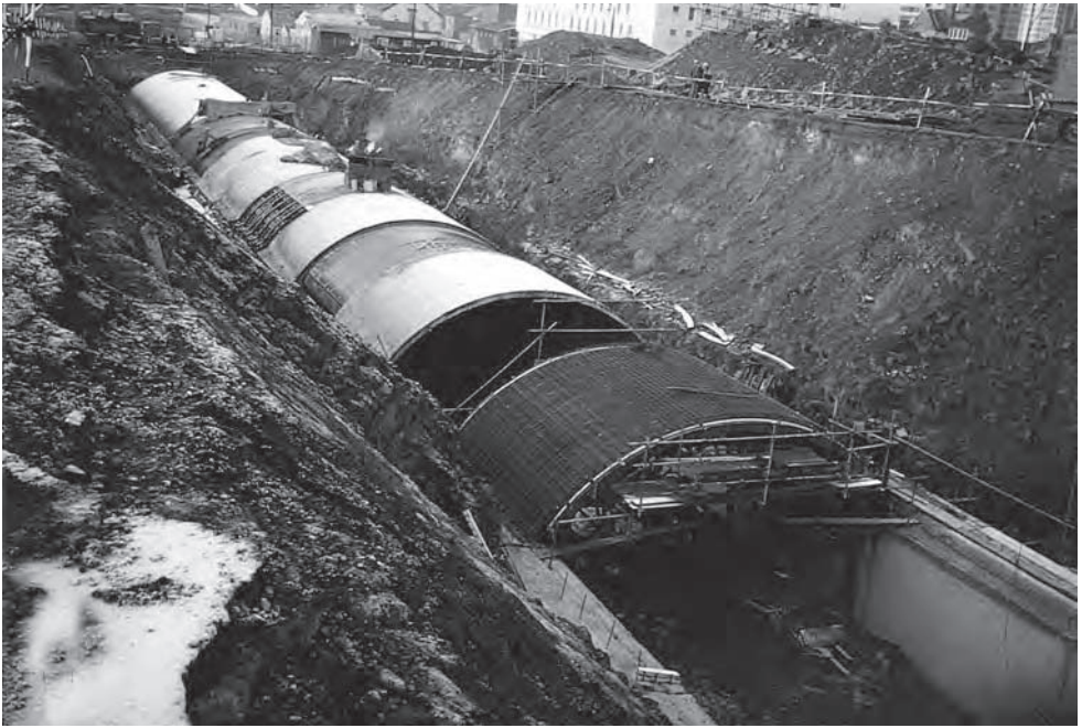
Figure 17.7 Byker Tunnel under construction (Photo: Robert Benaim)
