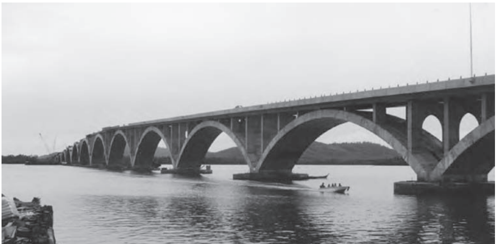
Figure 17.16 Bridge over Sungai Dinding (Photo: Benaim)
