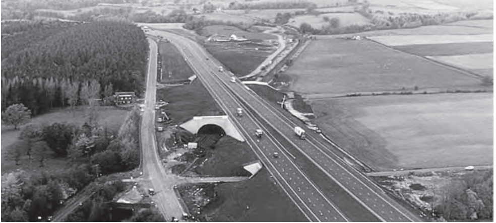
Figure 17.8 New Cowdens arch (Photo: Alister Lynn/Balfour Beatty Civil Engineering Ltd)
