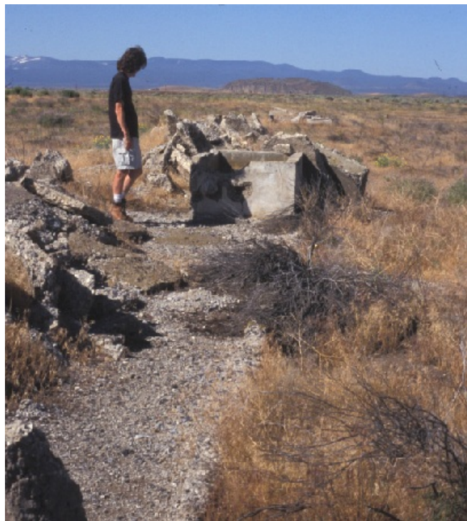
Figure 6.30. Remains of a latrine concrete slab in the evacuee residential area east of Tule Lake airport. Bulldozed concrete lying atop slab. Author photograph, June 2003.
