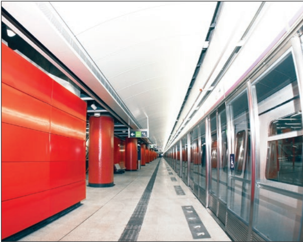
Figure 6.5 platform screen doors in use overseas
