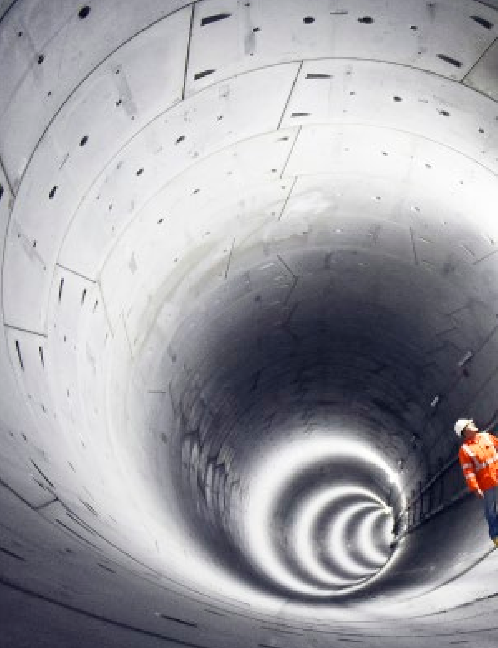
25 metres under Castle Hill in the city bound tunnel, May 2016
