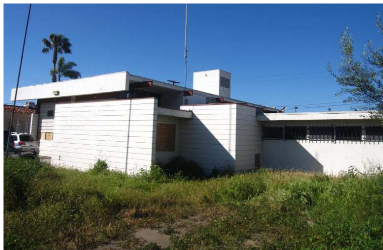
Former fire station, ca. 1960s (Source: Page & Turnbull)
