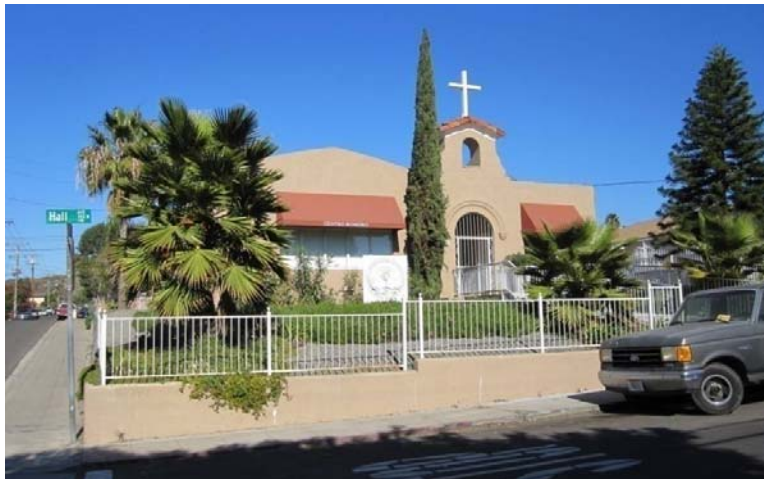
173 W. Hall Avenue, 1924, former San Ysidro Community Church designed by Louis Gill. (Source: Page & Turnbull, January 2010)
