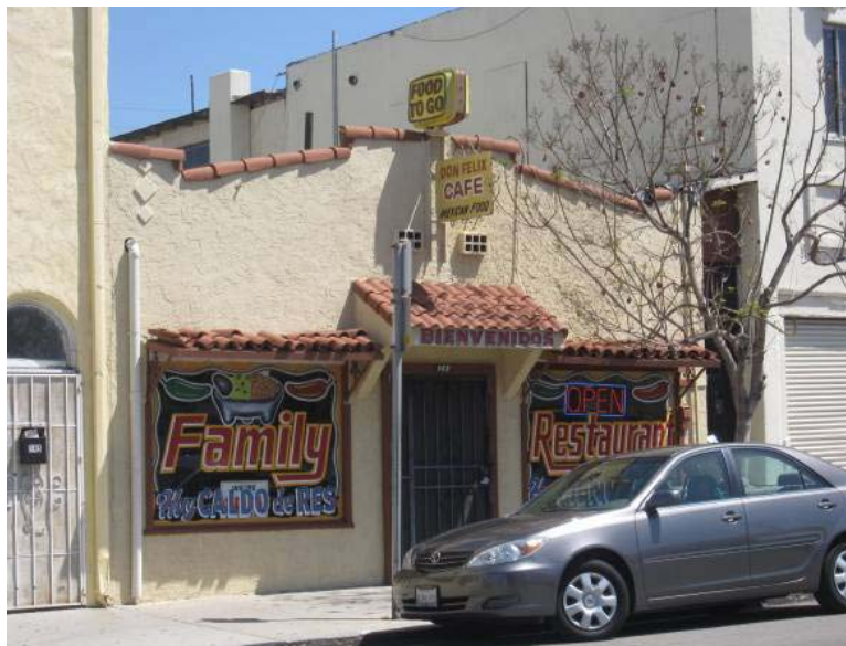
143 W. San Ysidro Boulevard, ca. 1920 (Source: Page & Turnbull, April 2010)
