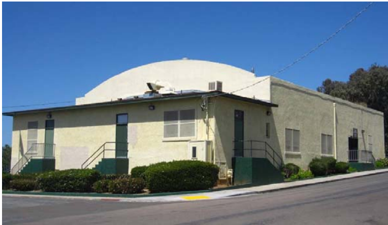
Civic and Recreation Center, 212 West Park Avenue, 1925 (Source: Page & Turnbull, April 2010)
