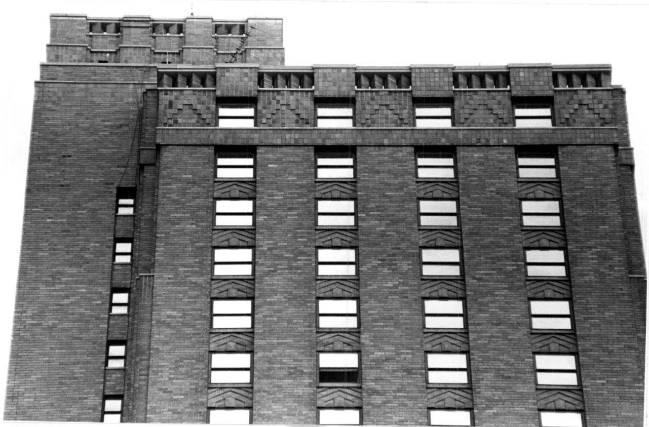
Downtown Athletic Club Building Roof details, West Street facade
