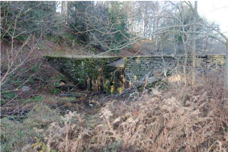
West Shore Road Dam
