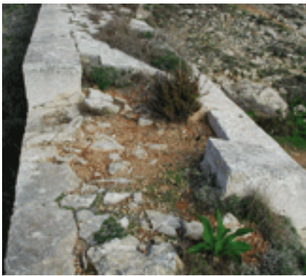
Above, top, Embrasure opening in parapet of Wied Musa Battery showing rusticated nature of masonry and use of ashlar quoins. Below, Parapet and gun platform of Wied Musa Battery (1715-16). This is one of the best preserved platforms of its type. Above, Superior slope of Ta' Kassisu entrenchment showing soil-bound rubble fill.
