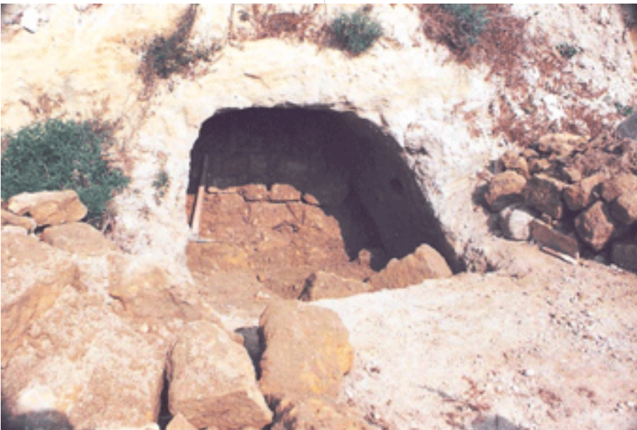
Below, Subterranean mine entrance as discovered in 1991 (photo by Mr. George Vella). Note the rough finish of the visible wall sections sealing off the mouth of the gallery.
