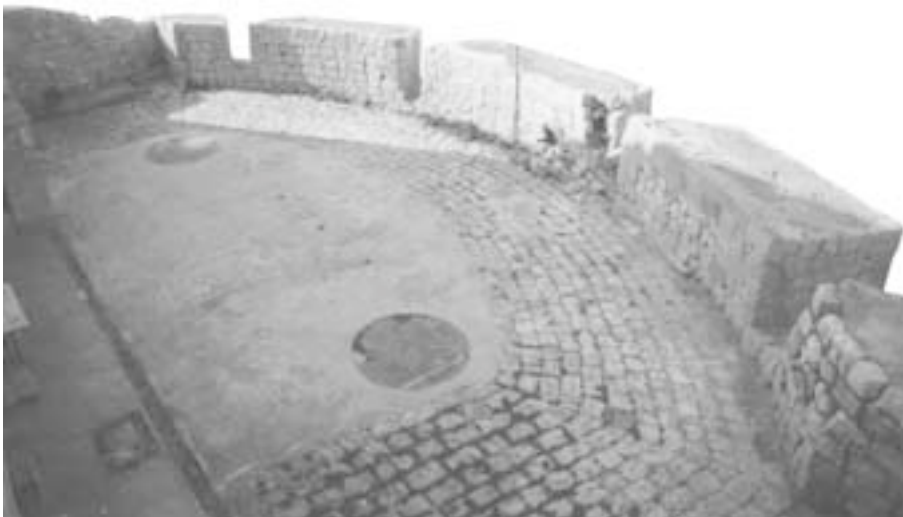
Above, top, Embrasure opening in parapet of Wied Musa Battery showing rusticated nature of masonry and use of ashlar quoins. Below, Parapet and gun platform of Wied Musa Battery (1715-16). This is one of the best preserved platforms of its type. Above, Superior slope of Ta' Kassisu entrenchment showing soil-bound rubble fill.
