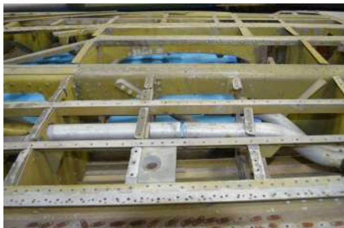
N13Y Radiator/Oil Cooling Tubing in Wings
