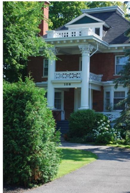
component of the porch such as a bracket, railing, post, baluster or column has deteriorated beyond repair, it should be replaced in the same style, material, and proportions.
