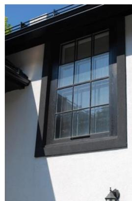
5. Retention of original fenestration pattern is encouraged. Where a new window opening is required, it should follow the rhythm and scale of the historic pattern.
