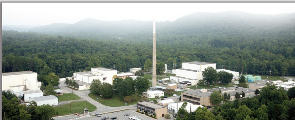
HFIR/REDC reactor/hot cell complex (ORNL)
