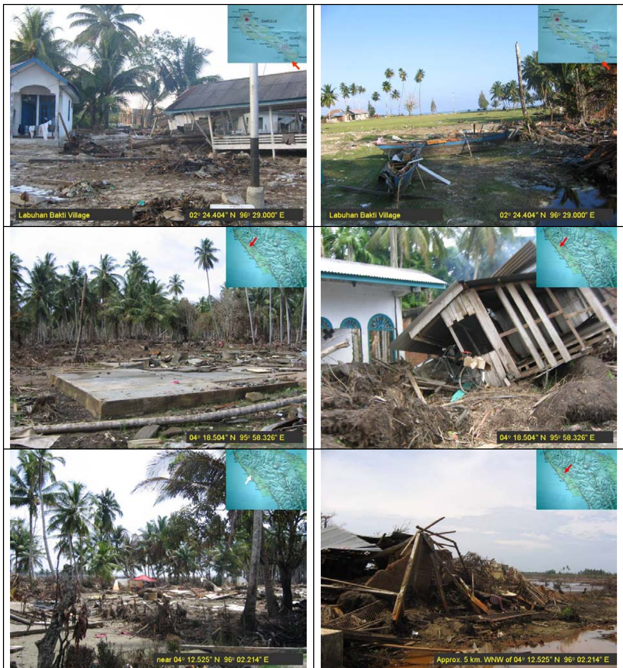
Figure 7: The typical damages and damage levels of tsunami on wooden structures.
