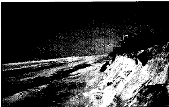
Highway 98 between Fort Walton Beach and Destin was destroyed by storm surge. Above(left) is an aerial view of highway 98 and above(right) is a close-up view of Highway 98.
