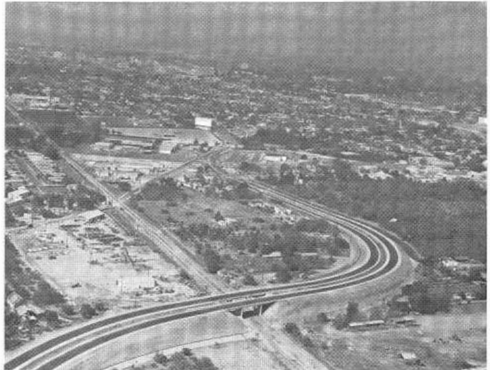
An aerial of a section of the new Almaden Expressway south of San Jose constructed by Santa Clara County under the Federal-aid Secondary Highway Program. Note the narrow railroad underpass on the old road at the left.
