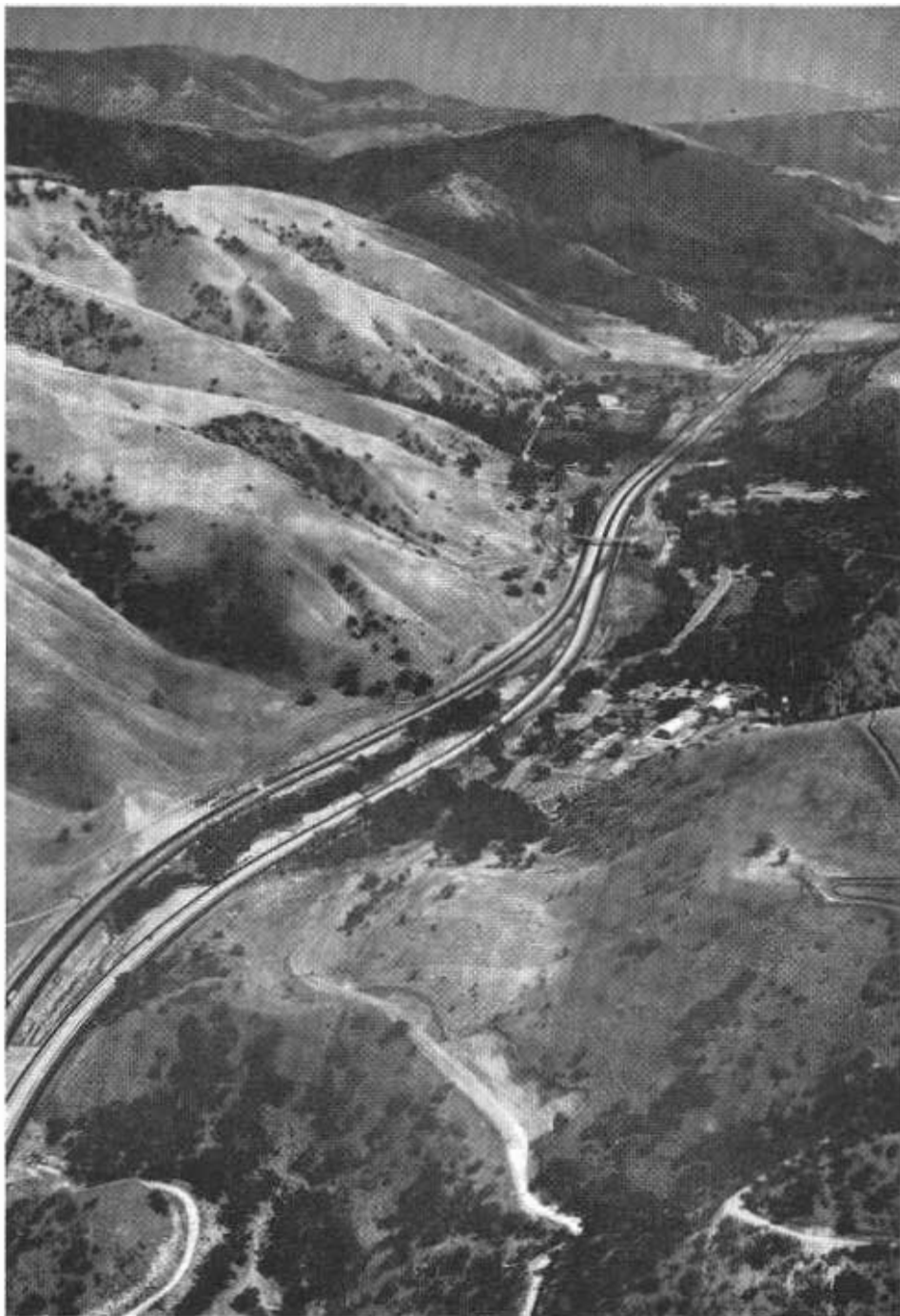
The view southward from the top of the grade with the Fort Tejon Interchange at the center of the picture.
