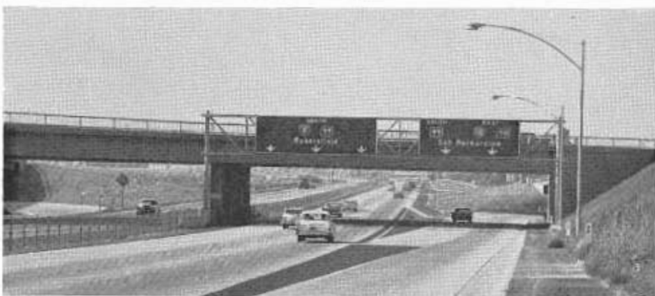
PHOTOS ABOVE—Sequence signing in advance of a freeway junction under crowded urban conditions.
