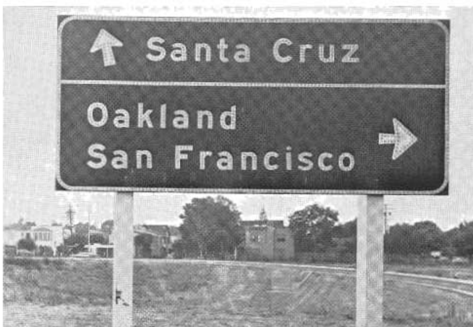
PHOTOS ABOVE—Guide signs include divider when they have destinations in different directions.
