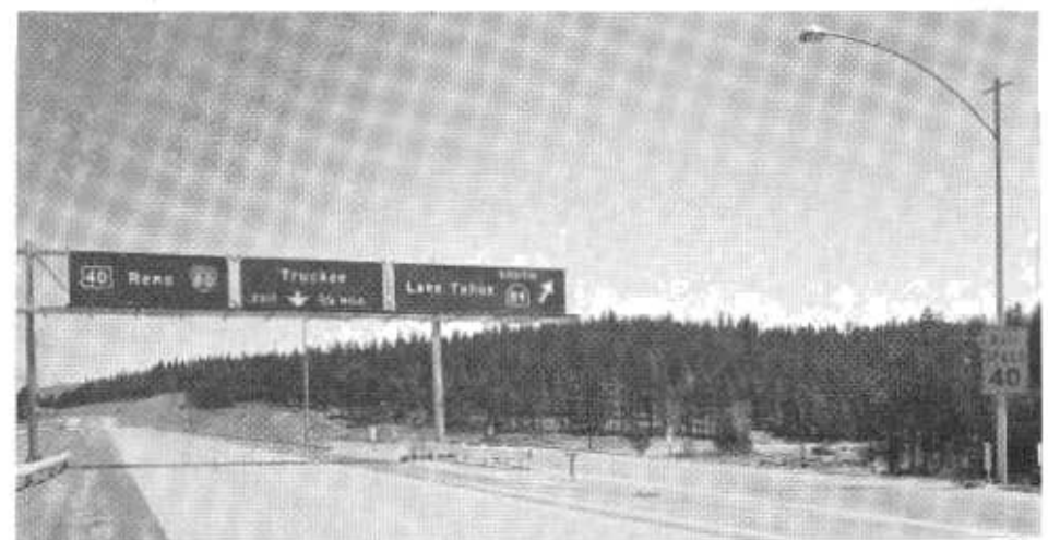
PHOTOS ABOVE—These signs give repeated notice of an important sign route turnoff.
