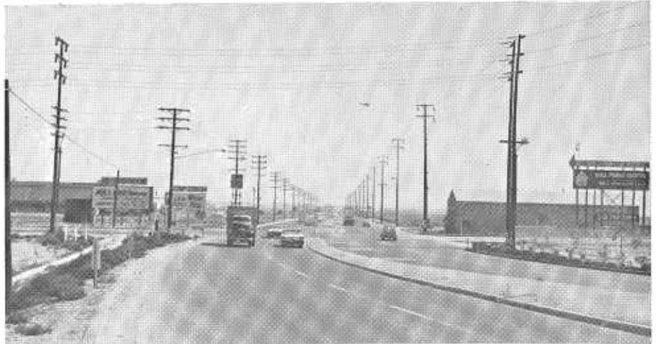
Harbor Boulevard (between the Cities of Santa Ana and Costa Mesa) was built cooperatively as a Federal Aid Secondary highway using the Arterial Highway Financing Plan.
