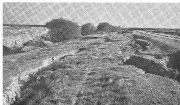
Plate 8. Shallow subsidence occasioned by a new abandoned irrigation ditch.
