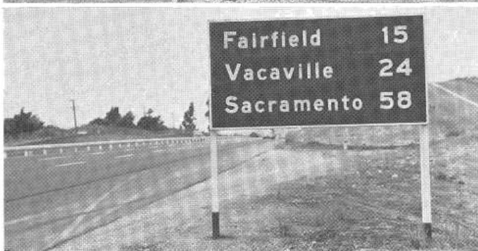
PHOTOS ABOVE—Reassurance signs are larger and reflectorized for easy nighttime as well as daytime reading.
