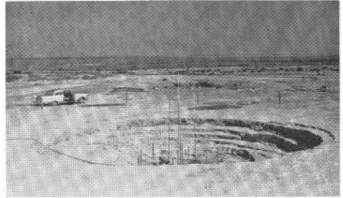
Plate 7. The Department of Water Resources subsidence test plot after six months of operation.
