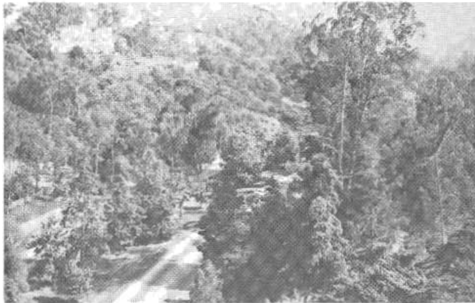
A view of the Cabrillo Freeway before clearing operations began.
