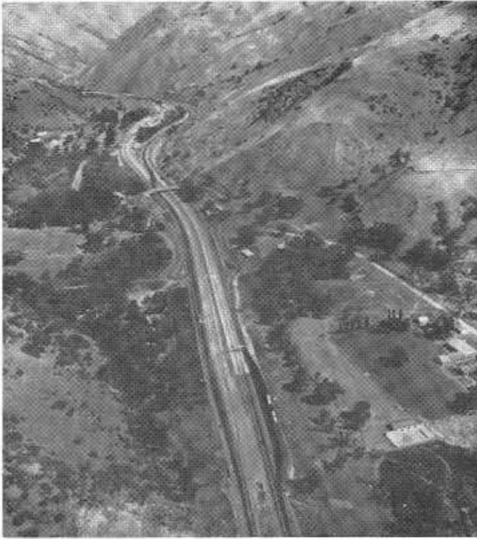
Looking north from the south end of the project toward Fort Tejon Overcrossing with Old Fort Tejon in left middleground of the picture.
