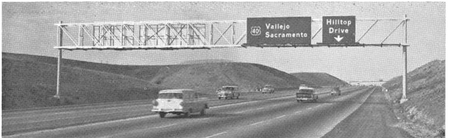
A sign bridge spanning both roadways of a modern freeway.
