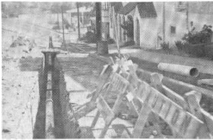
Water line relocation at Ninth and Ash Streets in San Diego.
