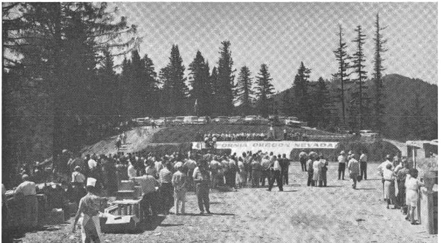
Some 500 people attended the groundbreaking ceremony which was preceded by an old-fashioned barbecue. The tunnel passes through the ridge about 450 feet directly below where the ceremony was held.
