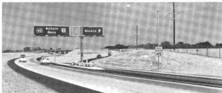
PHOTOS ABOVE—Approaching a turnoff to a community from a major rural freeway, the motorist is notified repeatedly.
