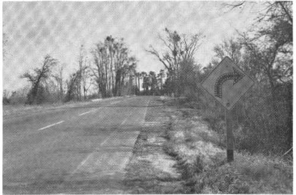
A diamond-shaped yellow sign indicates a warning; reflectorized arrow specifically warns of curve to right ahead.
