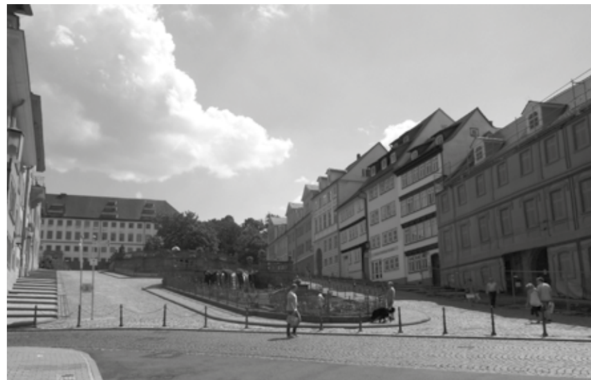
Fig. 4: Scene of Gotha town below the Friedenstern castle, with the house of Hiob Ludolf on the right, in which he worked on his Ethiopianist oeuvre (currently in renovation), 2014
