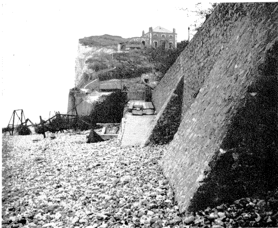
THE SEA-WALL AT PUYS, LOOKING EAST
