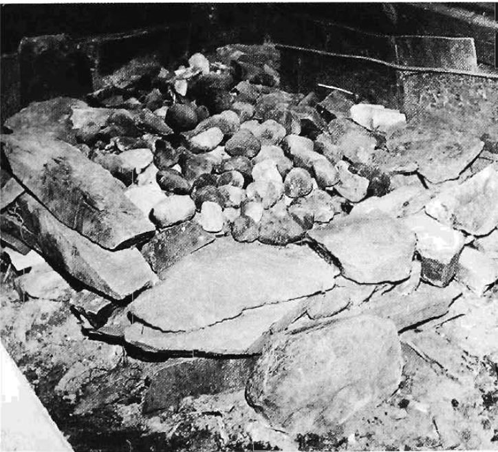
THE HYRYNKANGAS stove (above) is a traditional kiuas. The rocks and stone fragments over the fire chamber are supported by transverse beams and mantel, both made of stone. Above right, Albin Tikkanen, a Finnish immigrant, tends the fire in the savusauna he built in 1922. This is a modified kiuas with a rail mantel over the fire. At right the stone-covered oil barrel stove with a connecting stovepipe chimney is a "third generation" stove. The more sophisticated kiuas reduced by two to four hours the time needed to heat the sauna.
