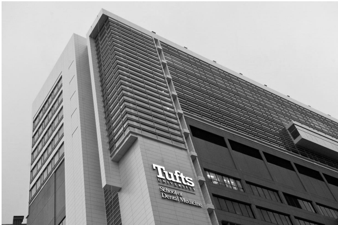
The Vertical Expansion Project at the Tufts University School of Dental Medicine in Boston, MA, September 17, 2009
