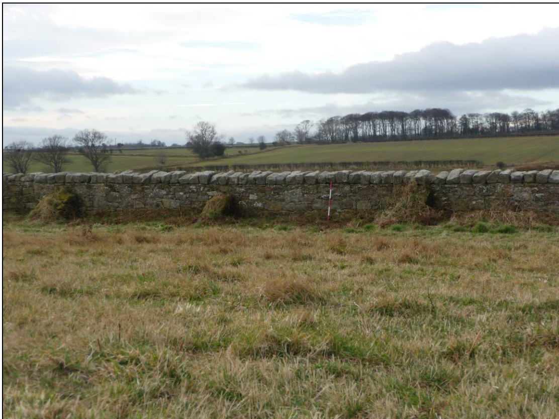
Plate 6. 18 th or 19 th century wall with buttresses (NT SMR 14595)
