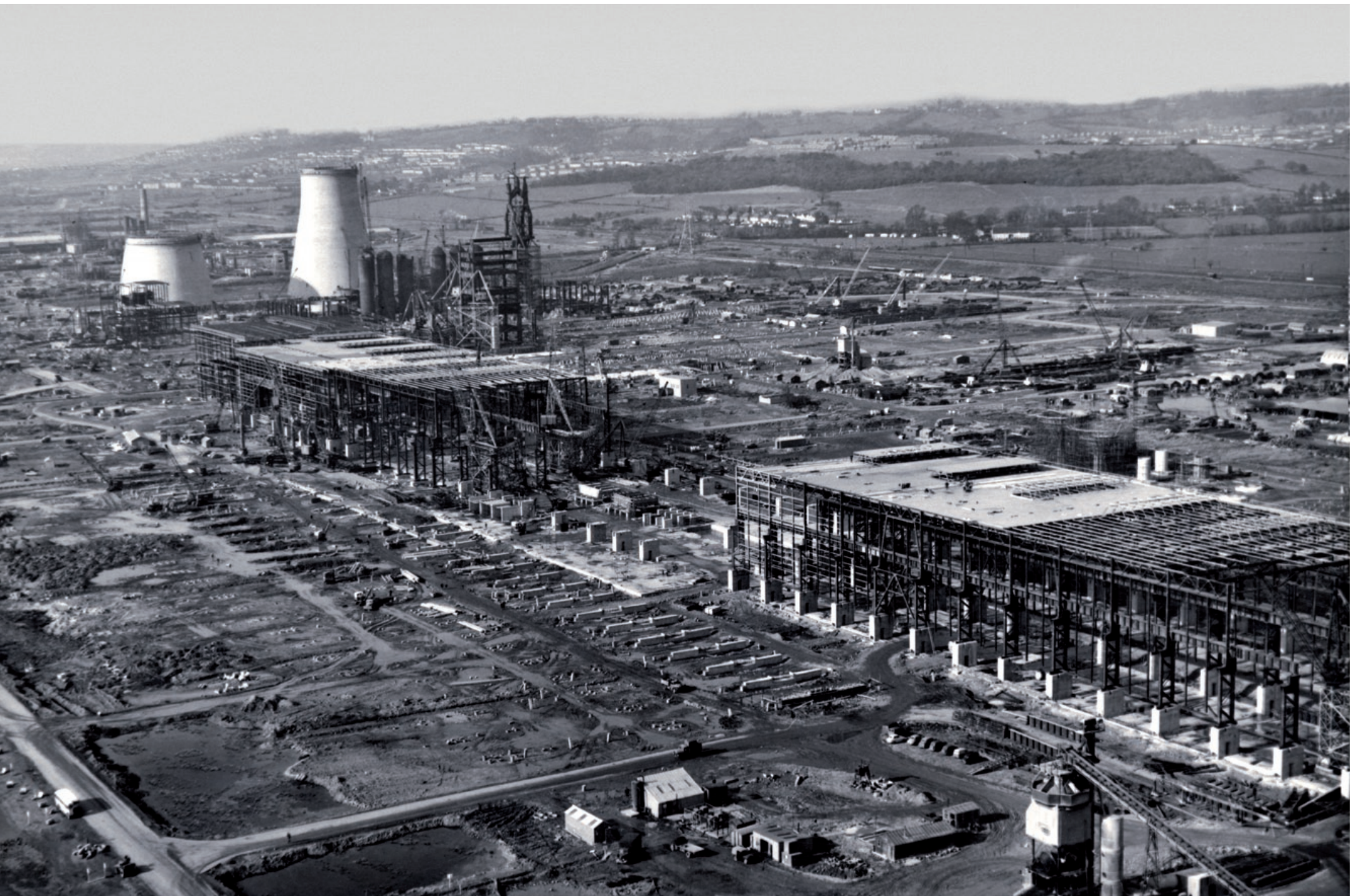
Spencer steelworks, Llanwern
