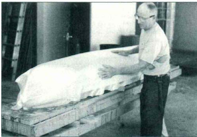
22. After you are satisfied with the sanding, give the bare wood a coat of epoxy. Let this dry, and sand it lightly—just enough to rough it up; don't sand through to the bare wood. Cut fiberglass cloth to length, and drape it over the clean hull. I smooth all the wrinkles out by hand before I wet out the cloth.
