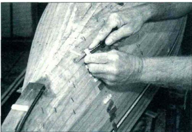
17. Use a tack puller to loosen the nails and staples. A pair of nippers will pull the nails out, and the staples usually just pop out with the tack puller.
