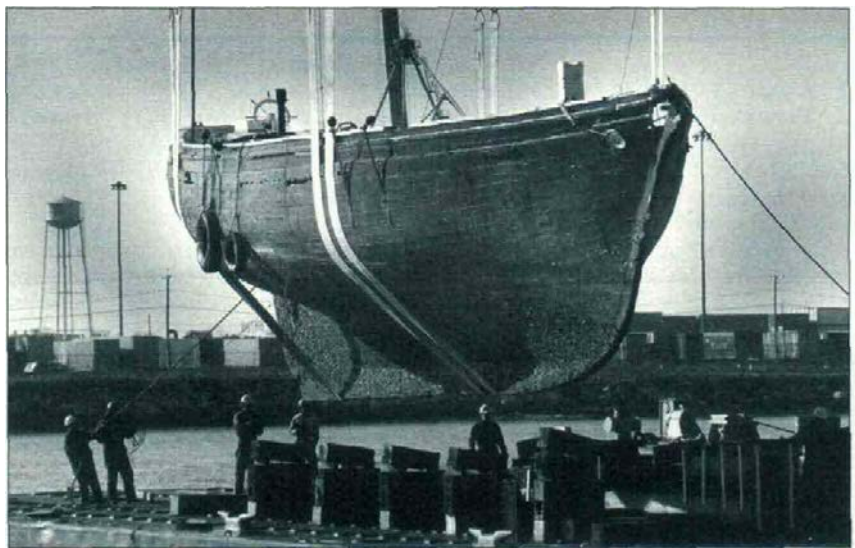
The Gloucester fishing schooner LETTIE G. HOWARD being lowered onto the barge where she will be restored.
