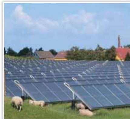
Denmark's Marstal site pipes 100% renewable heat.
