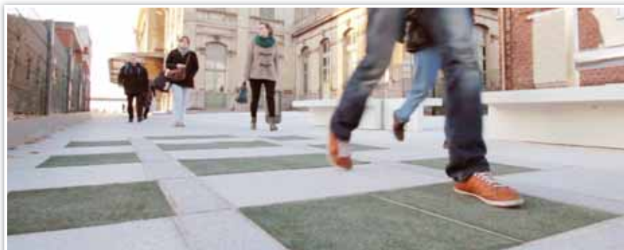
Tiles at the Saint-Omer, France, rail station capture energy to power lighting and charge visitors' mobile phones.
