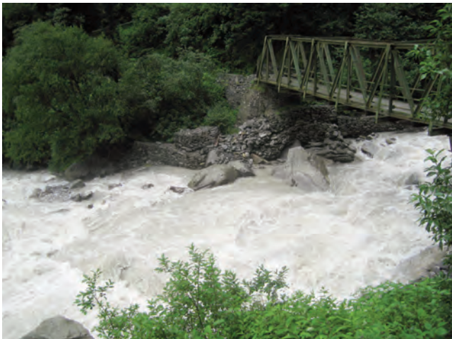
Bridge over Pushpavati
