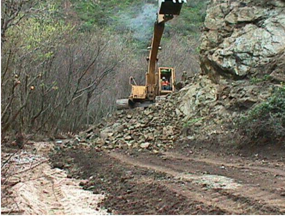
Driveway blocked at Garrapata
