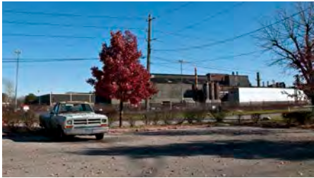
Site View 1: Navistar plant view looking east.
