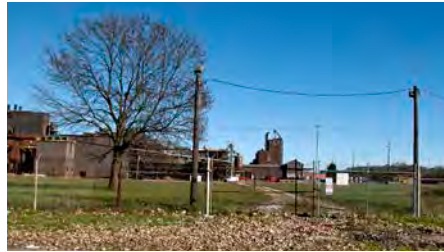
Site View 2: Navistar plant view looking east.
