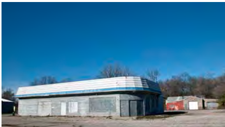
Neighborhood View 1: Abandoned retail along Brookville Road across from Navistar site.
