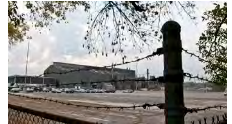
Site View 4: Navistar plant view looking southeast toward the foundry.
