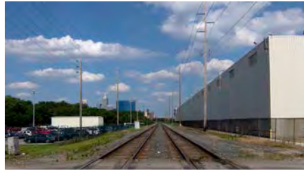
Site View 2: CSX main line looking east in General Motors site area.
