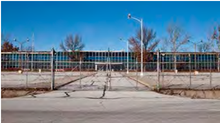
Site View 1: Ford/Visteon site view from English Avenue looking north.
