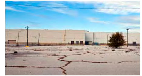
Site View 4: General Motors site looking north.
