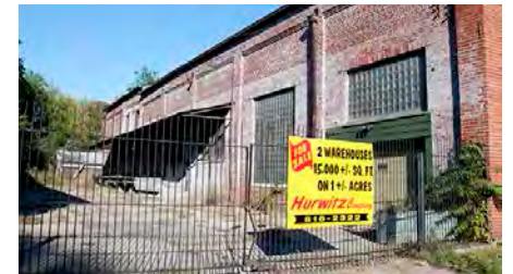
Neighborhood View 4: Older vacant industrial space in the area.
