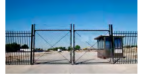
Site View 4: Chrysler Foundry site looking west.
