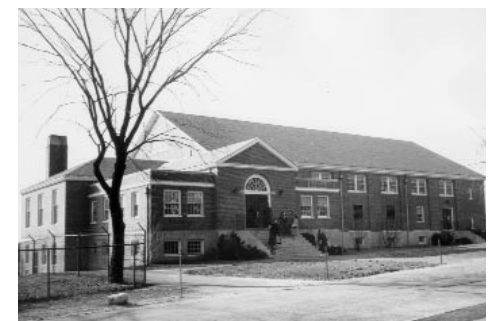
Jackson Gym, constructed in 1948, later became part of a complex of buildings including Alumnae Hall and the Aidekman Arts Center.
