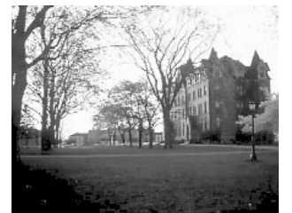
West Hall, built in 1872, is the oldest dorm in continuous use.
