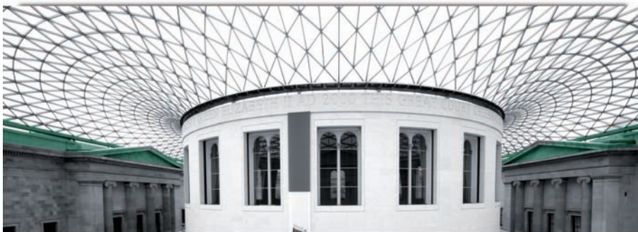
Figure 4.24: Roof over the Great Court of the British Museum, London, Foster+Partners, 2000.
