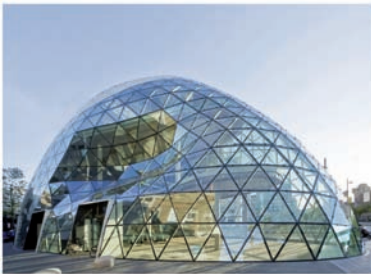
Figure 1.19: Skin - structure and facade of the 18 Septemberplein in Eindhoven, Netherlands, designed by M.Fuksas, roof structure by Knippers Helbig, finished in 2008.
