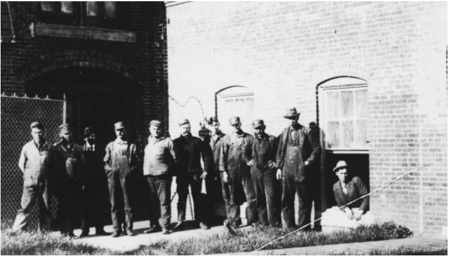
SHIFT WORKERS AT VEAZIE HYDRO (EARLY 1900's)
