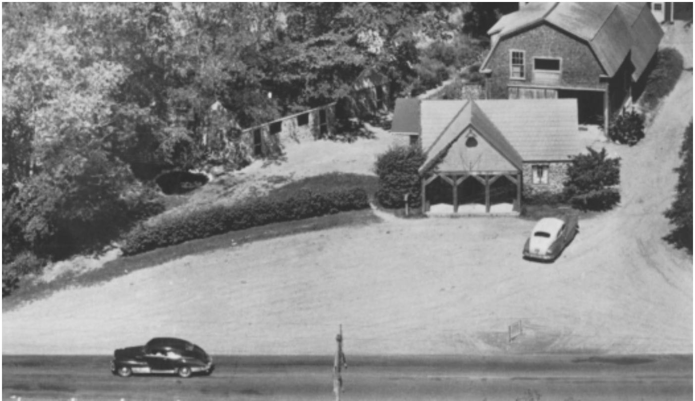
Building in center was used as the ice cream parlor.
