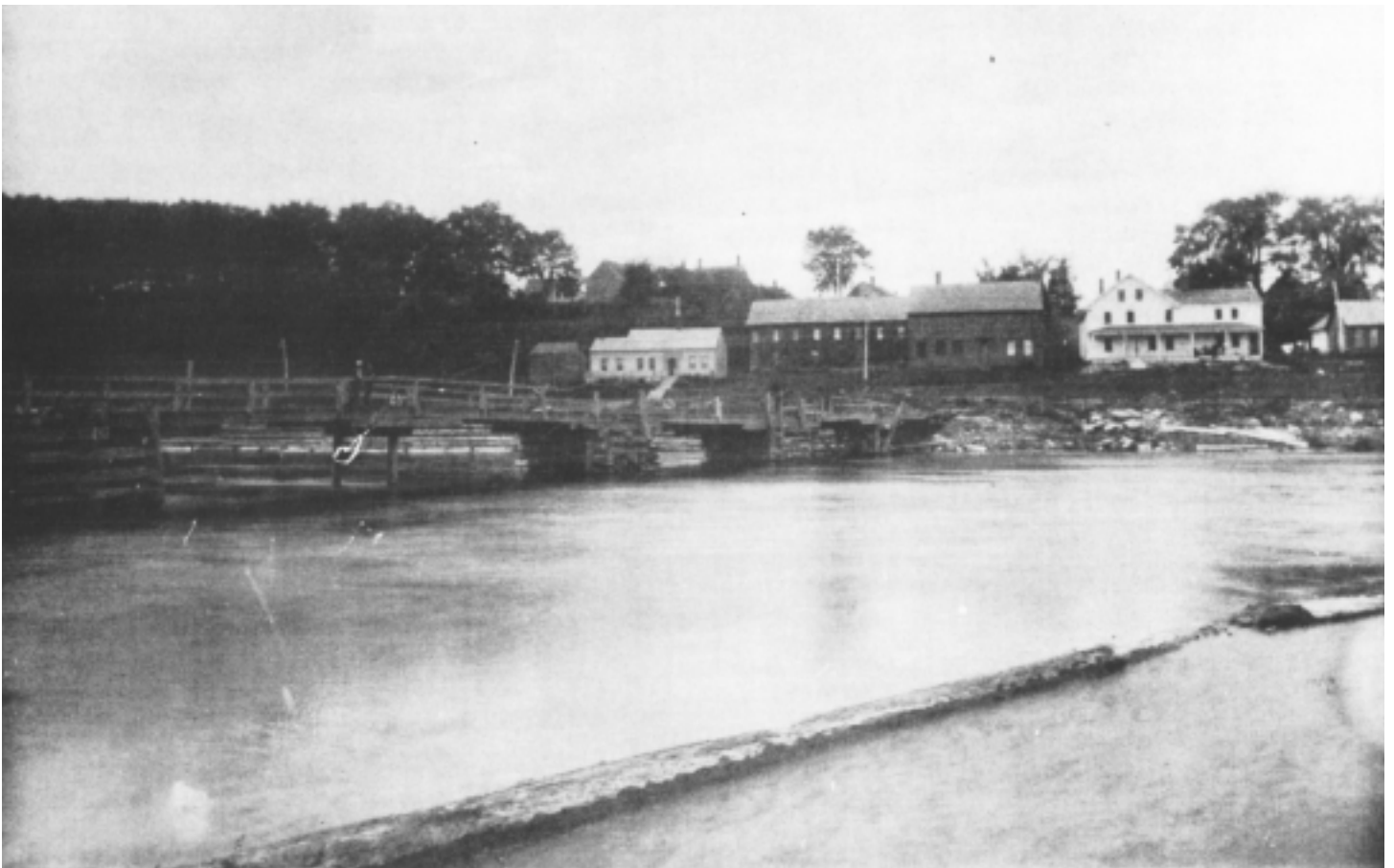
LATE 1800'S - Taken from the Old Wing Dam, showing the bridge to the lumber mill, and the mill company houses, on the shore above the power station.
