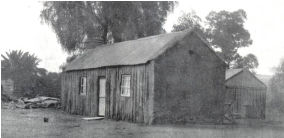
Myrtle Cottage was typical of housing in the town at the time of Flynn's first visit.
