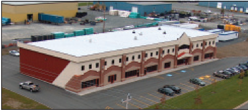
Cahill Instrumentation, 2 Southern Cross Road Photo: Sky-Shots Aerial Photography
