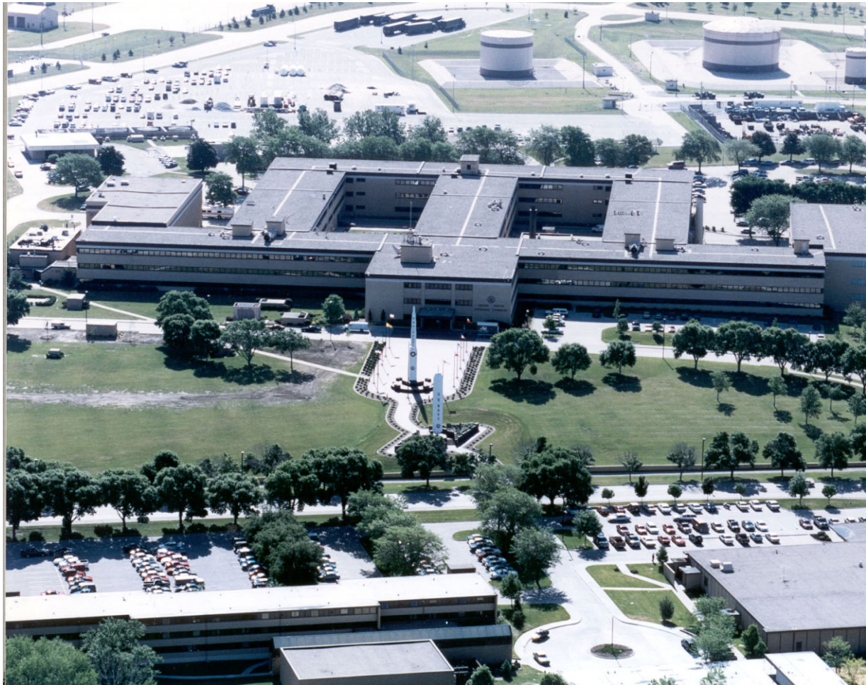
Headquarters USSTRATCOM, Curtis E. LeMay Building
