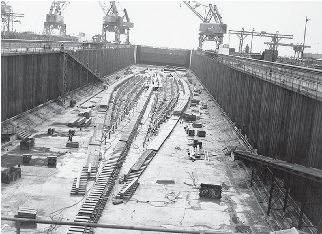
Keel for the first Supercarrier, USS United States, 1949
