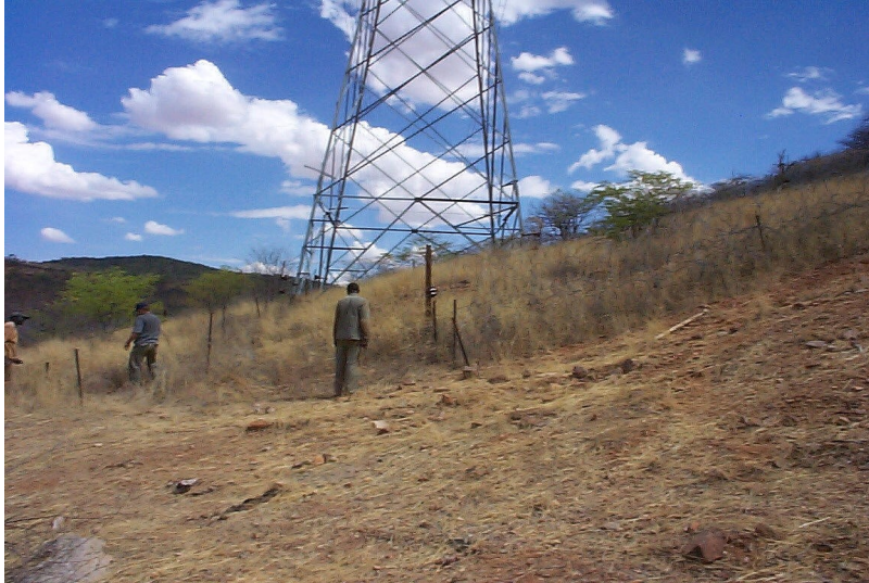
Pylon # 3. Note the steep slope.
