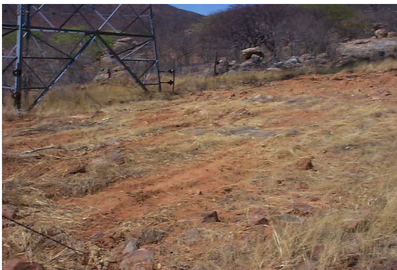
The final result of clearing pylon # 1.
