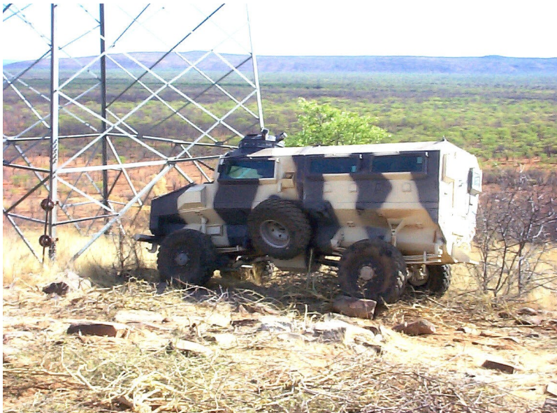
The 1 st pylon being worked. Note the vegetation.
