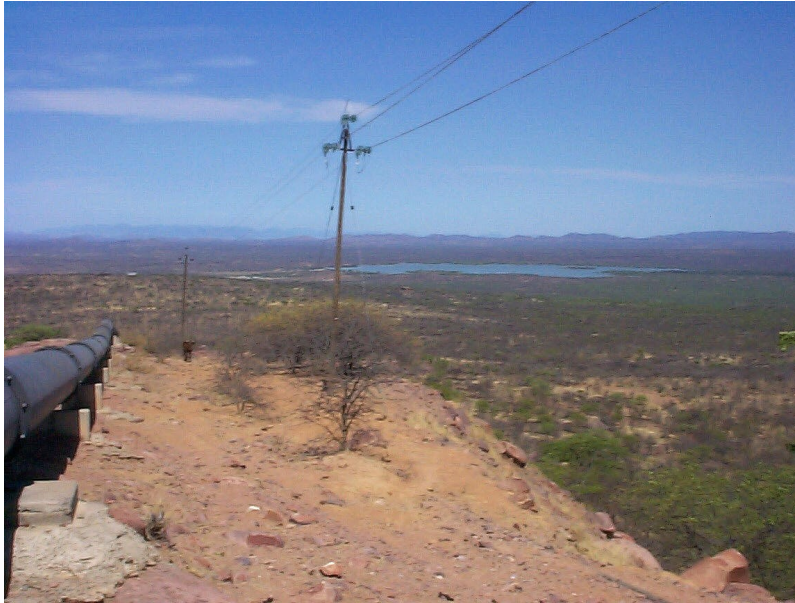
The Ruacana dam that feeds the hydro-electric plant.
