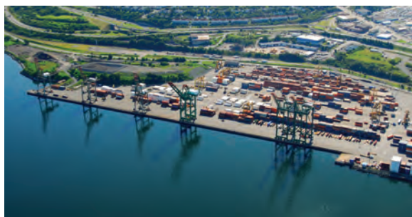
Fairview Cove container terminal
